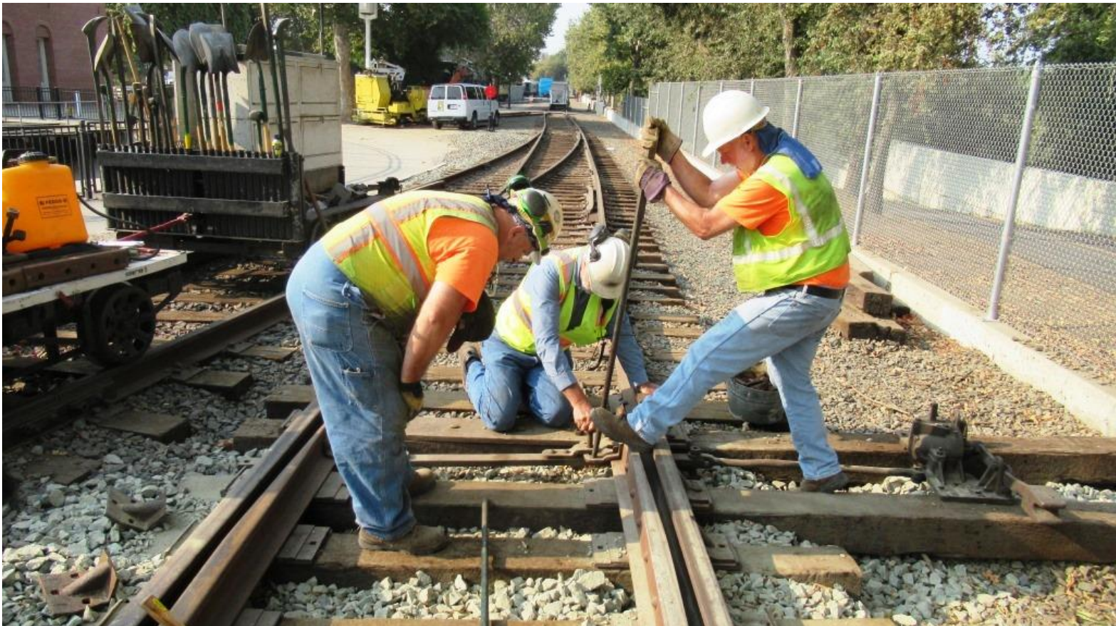
Mike F., Alan, and Mike M. begin adjusting the connecting rod's placement on the transit clip
