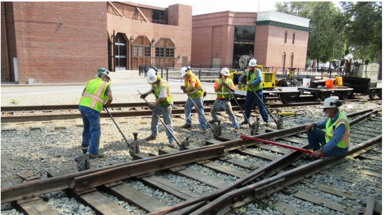
Team Track-Raise: Alan monitors the track-level as Ed, Matt, Bill, Mike M., and Weston all crank on the track-jacks in unison
