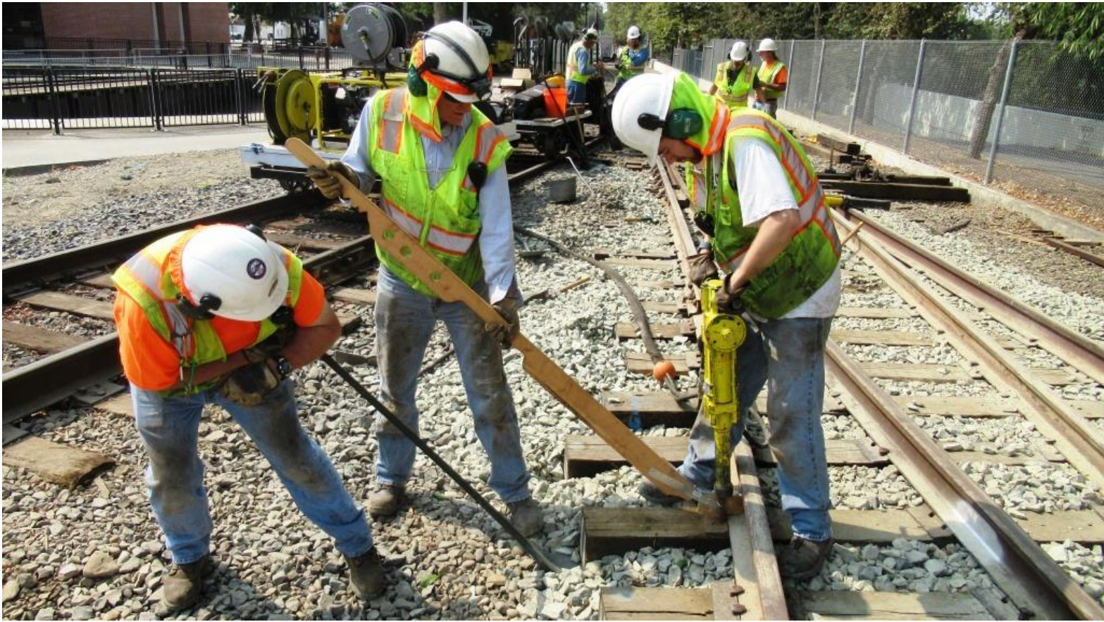
Bill nips as Steve uses the Steve-Tool to set a spike for Matt to drive with the hydraulic spike-driver
