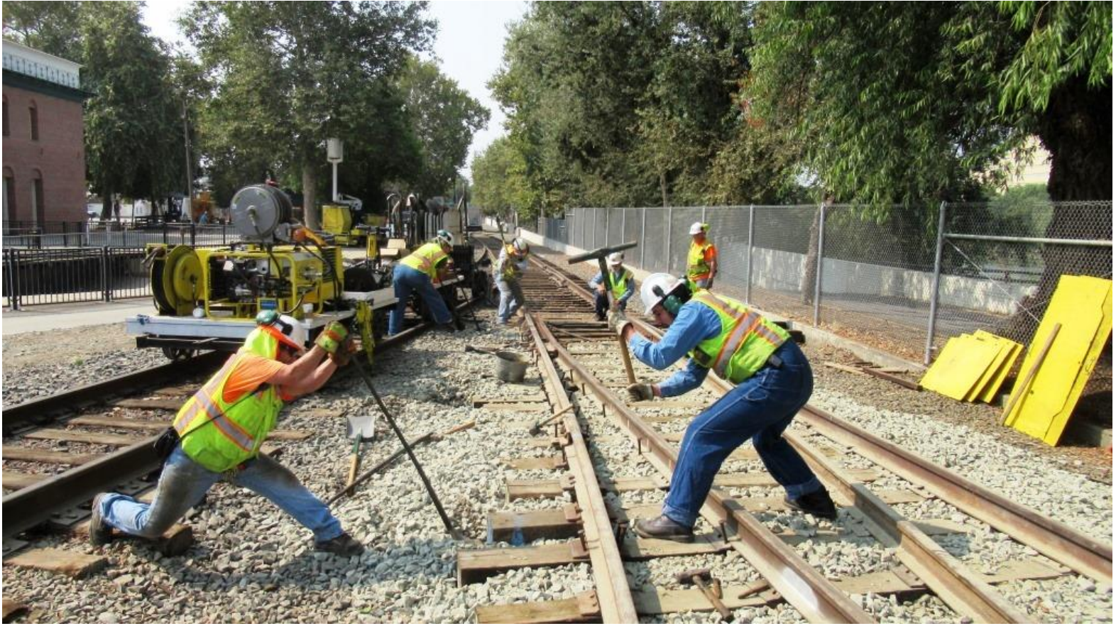
The insanity spreads: now Weston takes up the spike maul as Joe nips-up the tie
