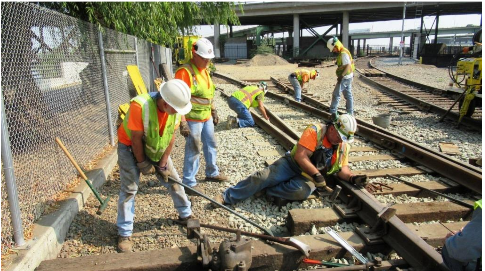
Mike M. nips the tie as Mike F. sets spikes on one of the rattle bracket plates
