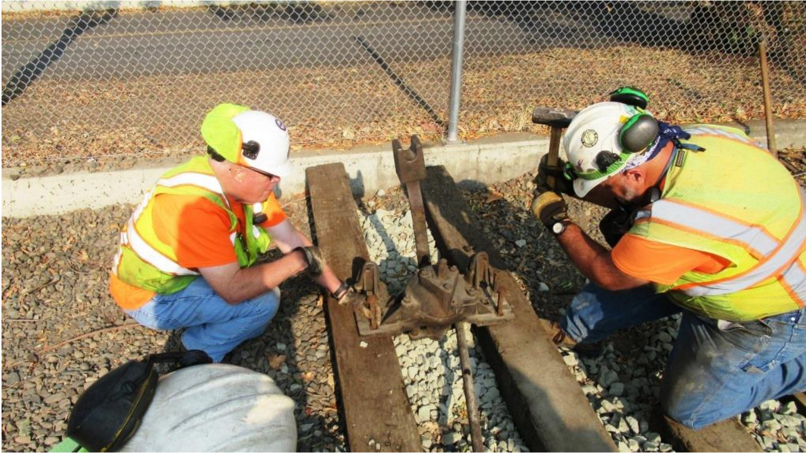
Bill and Mike F. tack-down the switch machine as they begin the adjustment process
