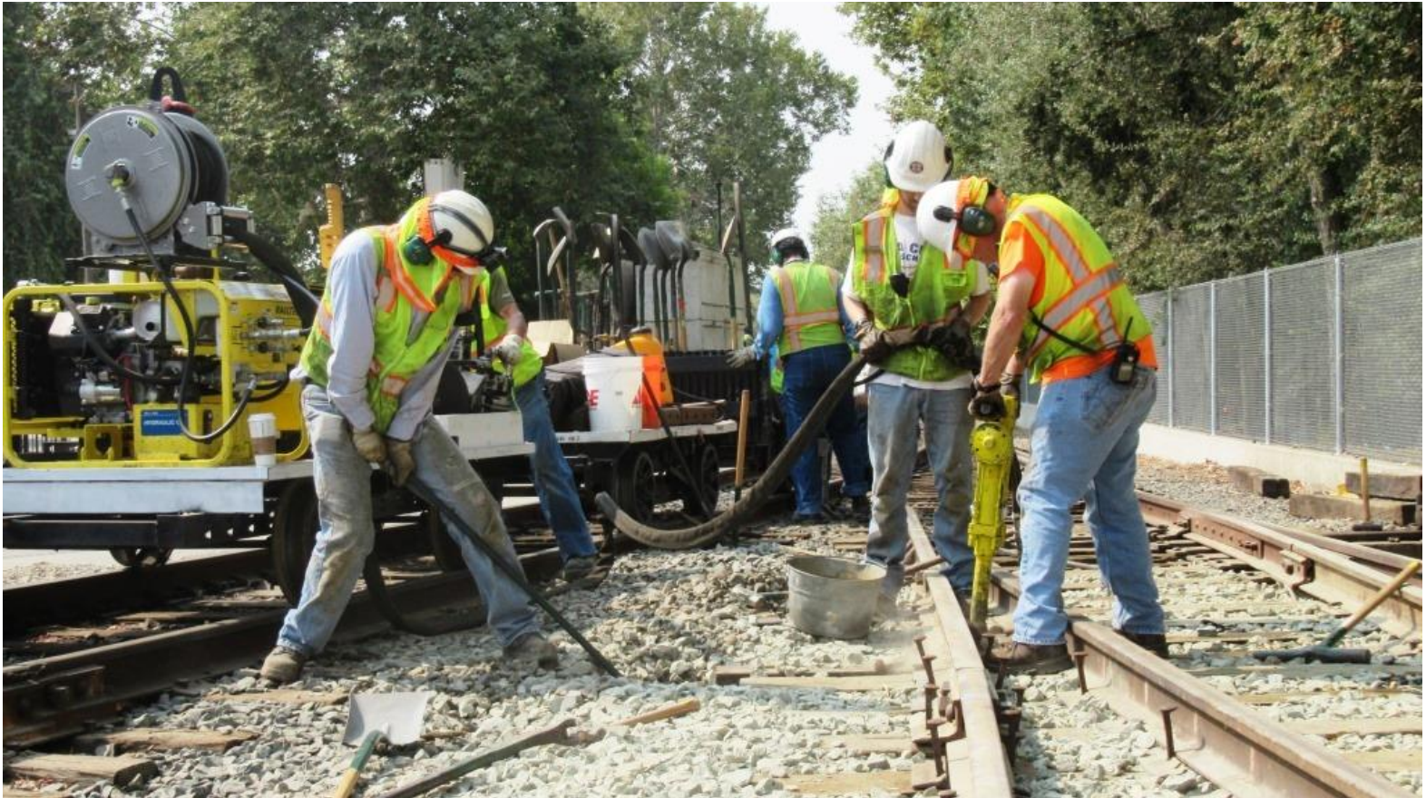
Steve nips-up the tie as Bill drives spikes with the hydraulic spike-driver
