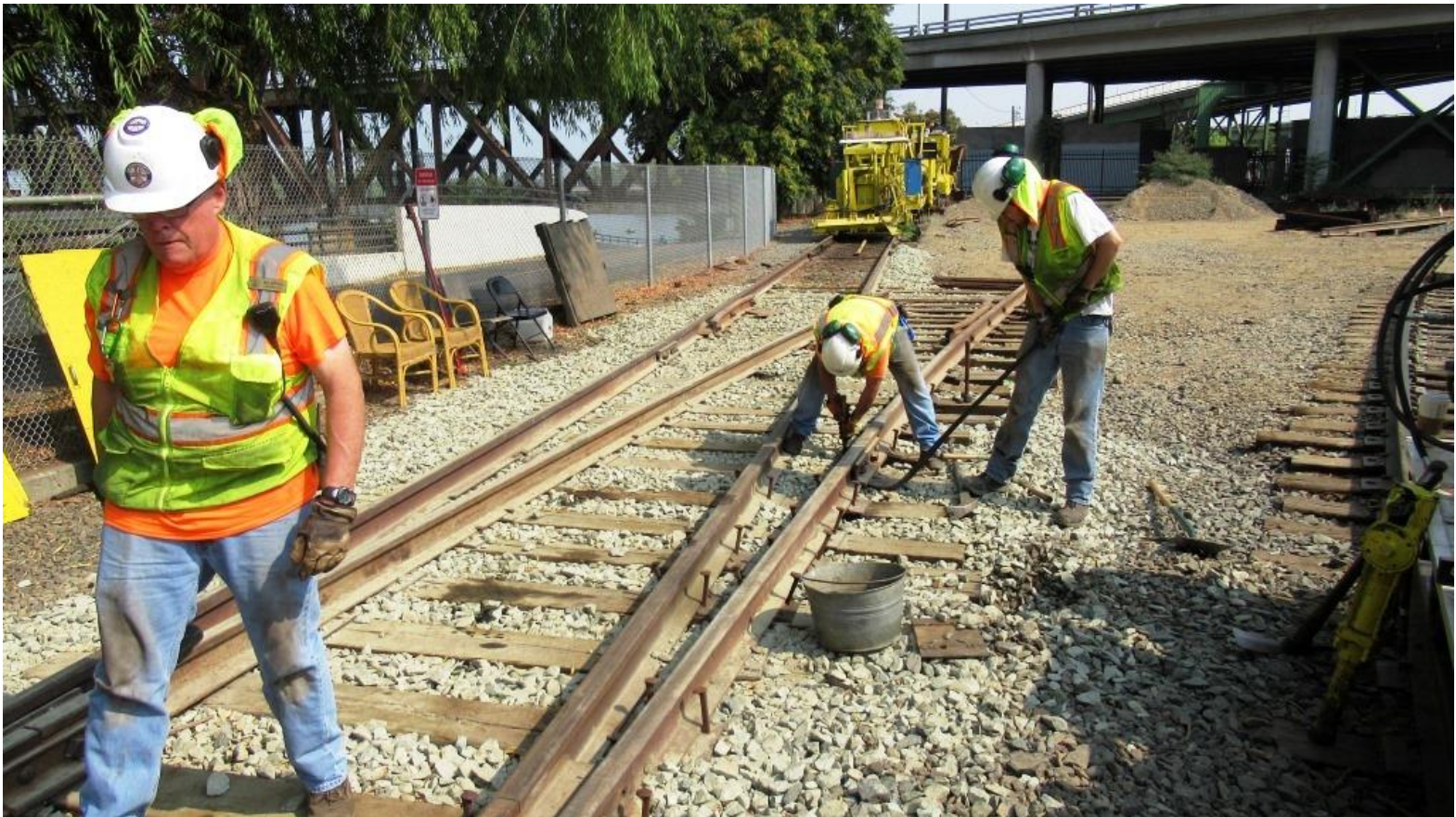
Meanwhile, Joe and Matt have set spikes along the diverging rail and closure rail
