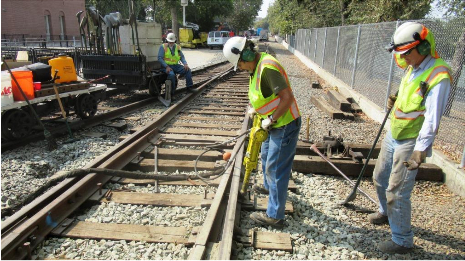
Ed brings sanity back to the operation by deploying the hydraulic spike driver
