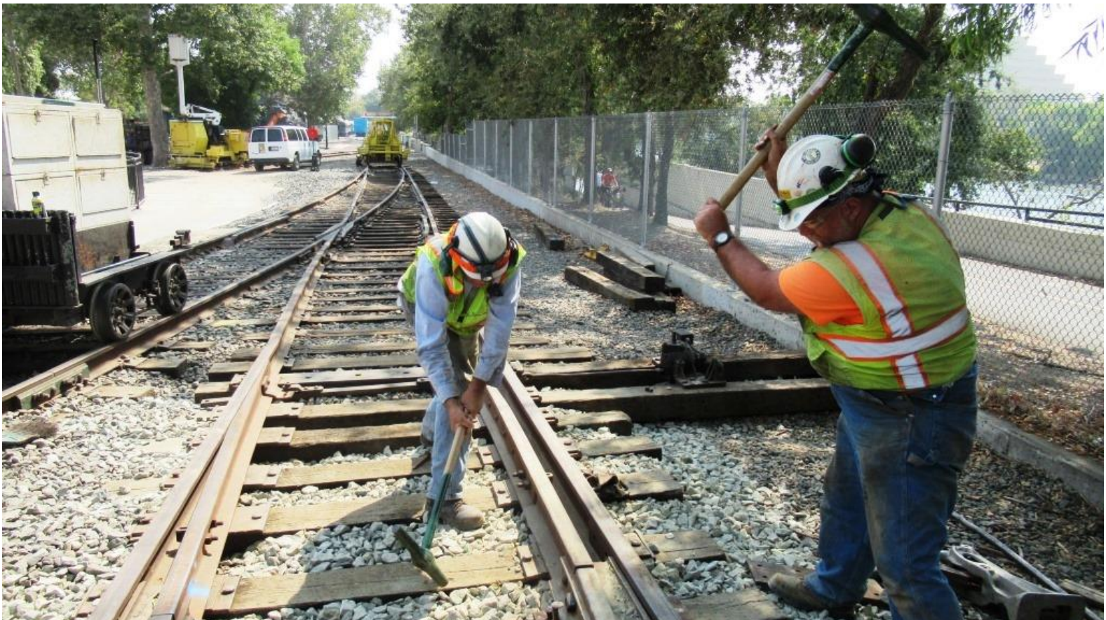
Steve and Mike F. do a little tandem spike-driving on the very last spike to be driven on the project
