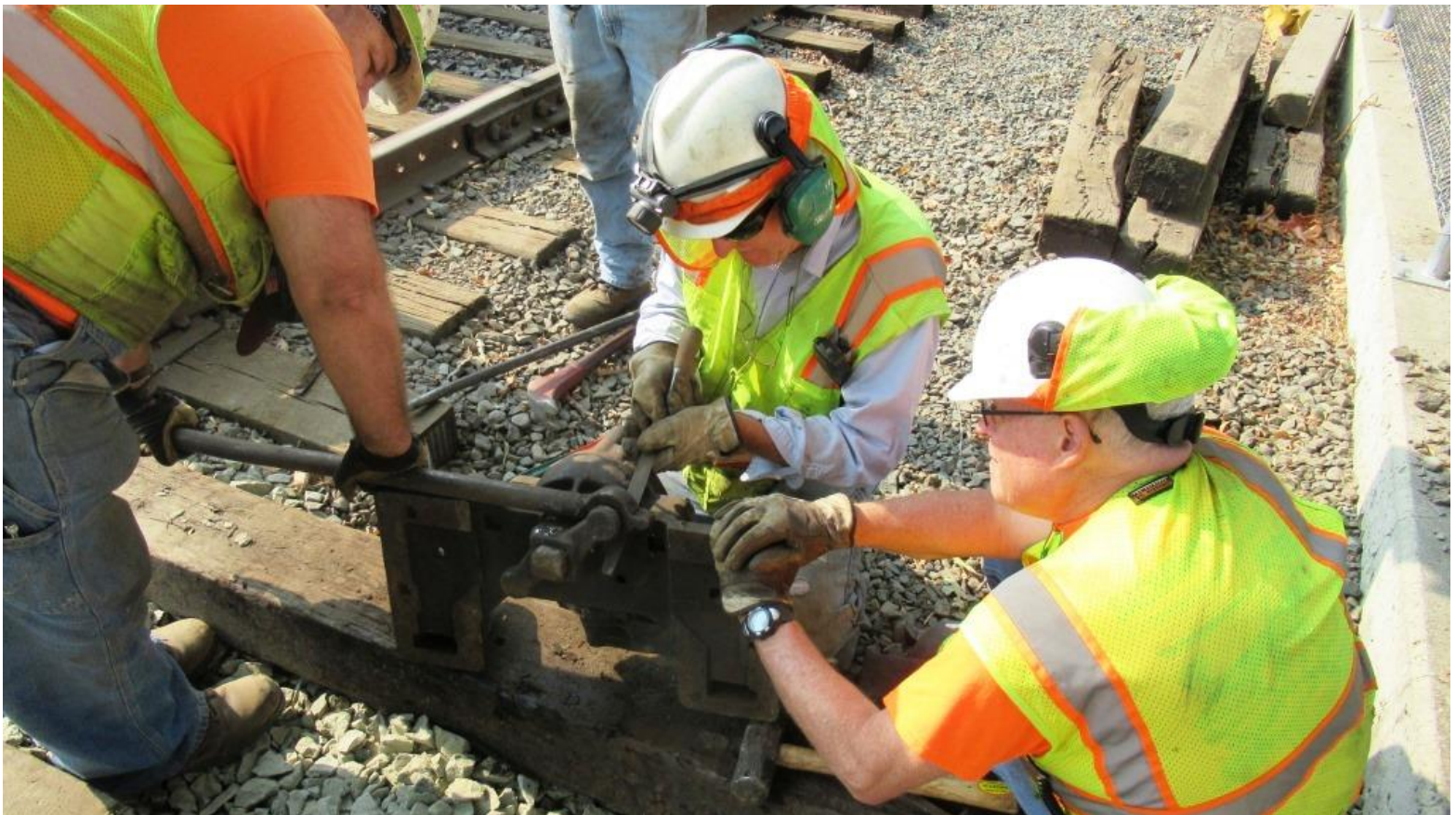
Steve uses a file to file down some protruding metal blocking the removal of the control rod
