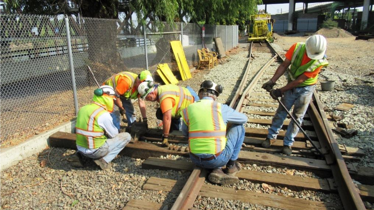
Mike M. levers over the points so that Steve, Bill, Mike F., and Alan can set the final placement of the machine
