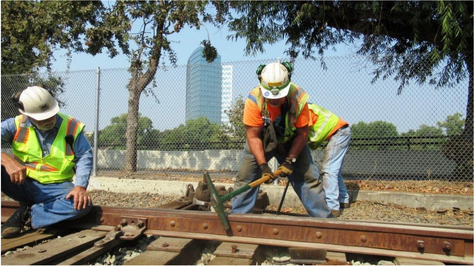
Mike F. now interprets old fashioned, track-gang railroading by driving the spikes by hand
