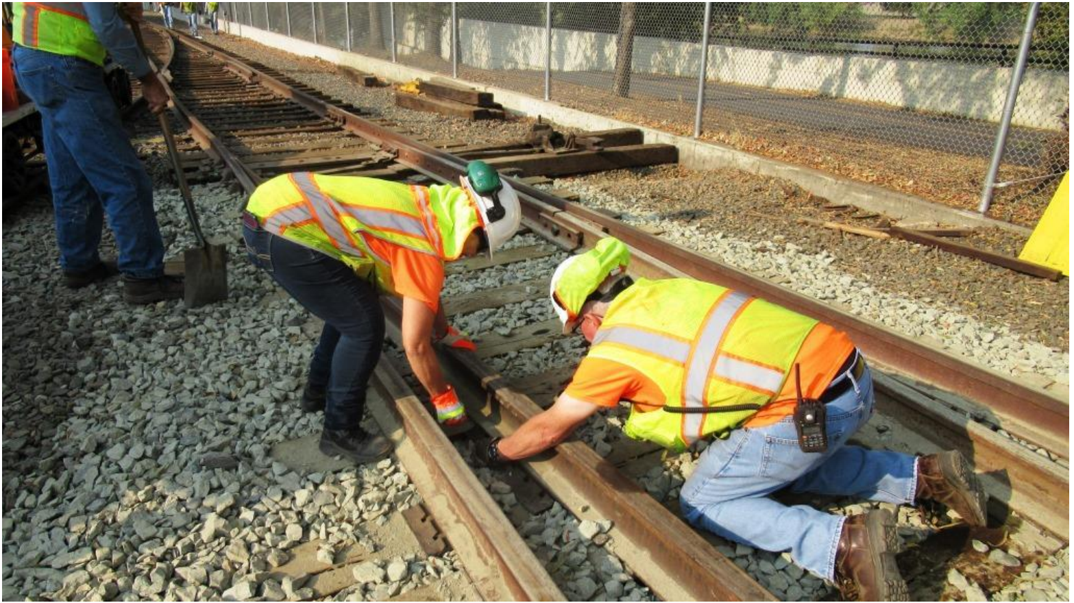
Pam and Bill place a plate under the closure rail
