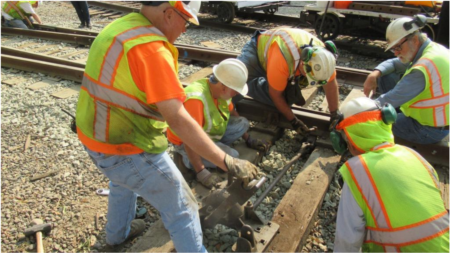
With the control rod now in the correct position, it can be hooked up to the connecting rod
